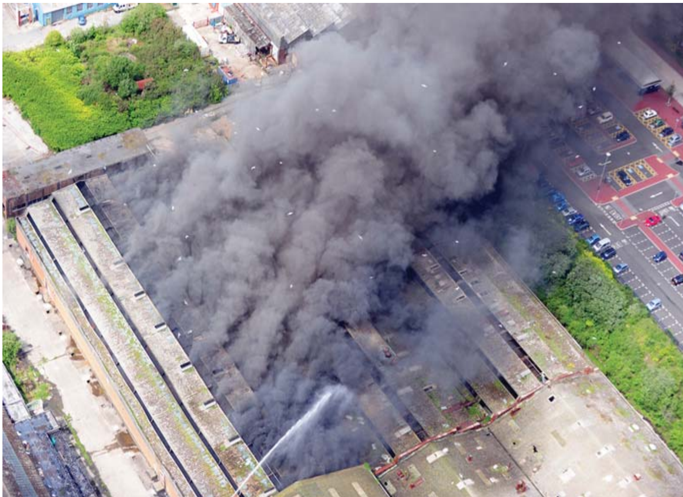
Photograph 2 – Fire at a depot in Swansea in June 2011 where tyre wastes were stored led to a major incident that lasted several weeks, threatened the evacuation of thousands of nearby residents, and cost the local authority and emergency services about £1.5 million.
