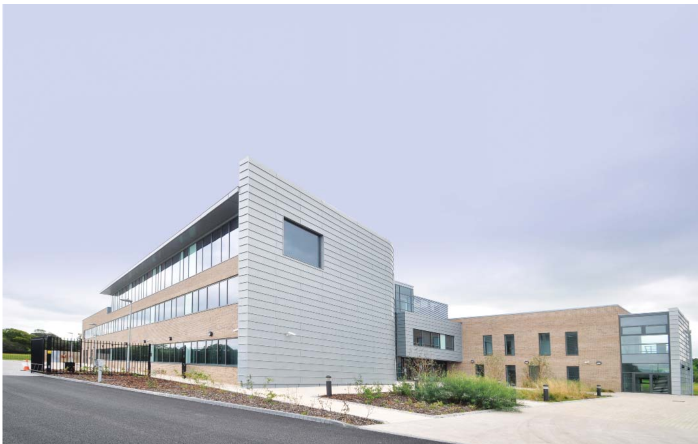
Photograph 1 – The Welsh Government and Dyfed Powys Police Force have built a new bespoke Strategic Coordination Centre in Carmarthen, one of three such centres in Wales.
